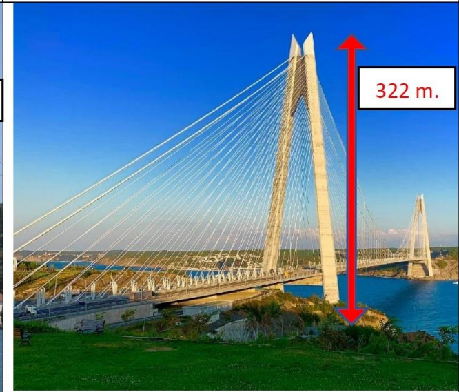
Fig.1d. The Yavuz Sultan Selim Bridge.
