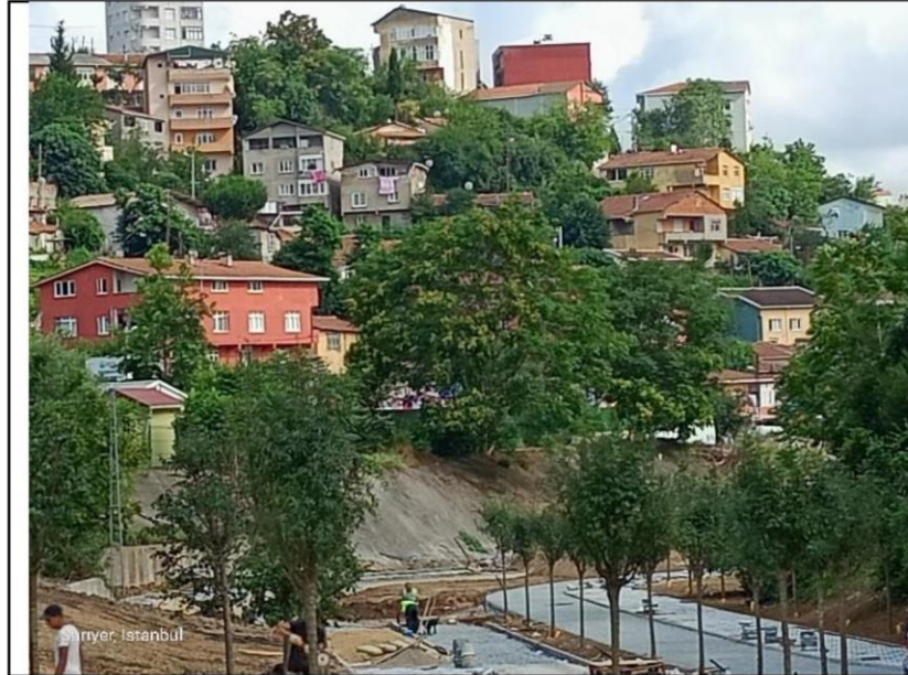
Fig.1. Housing near Site 5.
